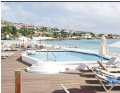
Pool deck with location of new beach bar in the background
